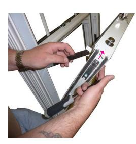
Slide restrictor arm upwards to remove from channel. Repeat the sequence on the opposite side of the window.
