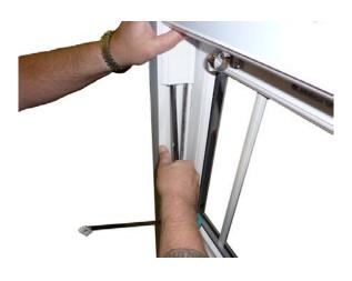
Use a screwdriver or similar to carefully prise the clip fit sash stop from it's location groove.
