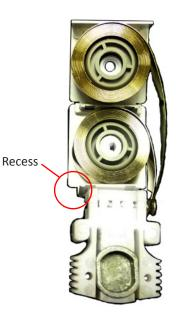
When fitting the new shoe and spring retainer ensure the small recess is at the bottom, failure to do so will affect the operation of the sash.
