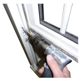
Remove the screws securing the springs
