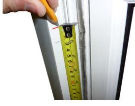
Carefully measure 20mm up from the pencil line and mark the outer frame
